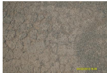
Location 2 – Crocodile cracks
