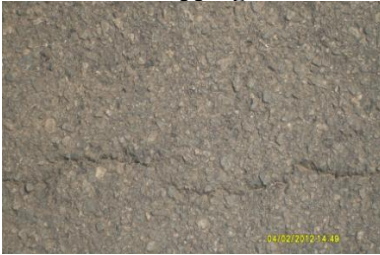
Location 5 - Longitudinal crack
