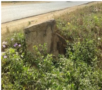
Culvert Inlet Overgrown
