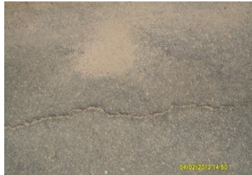
Location 4 – Longitudinal crack
