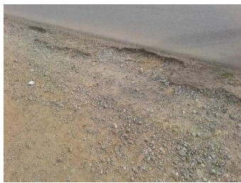
(a) Edge and Shoulder Damage
