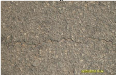
Location 7 - Longitudinal crack
