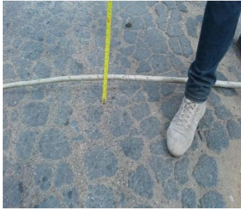
Rutting between CH. 3+000 and CH. 3+500
