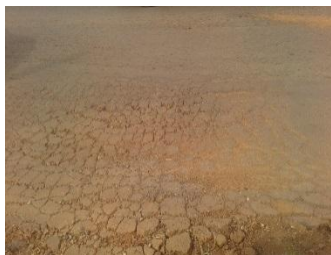
(c) Alligator Cracks
