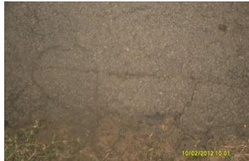
Location 10 –Longitudinal and Transverse Cracks
